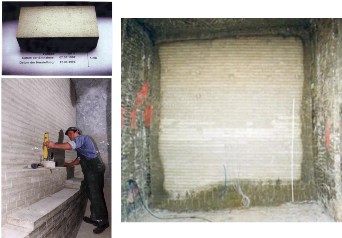
Figure 1.13 Single bentonite block, emplacement of blocks (both left) and sealing element before dismantling (right)
