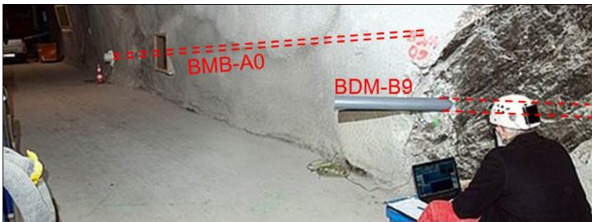
Figure 8.20 In-situ setup for the feasibility tests between boreholes BDM-B9 and BMB-A0
