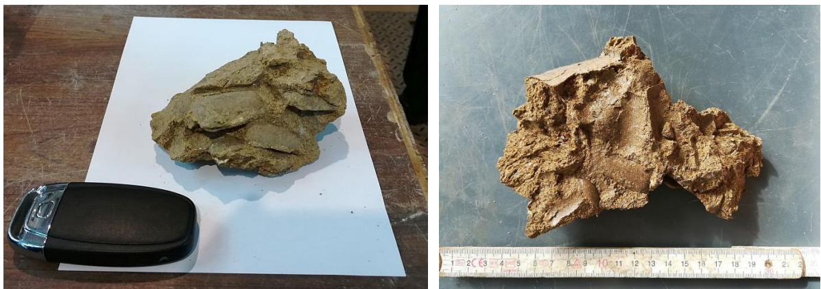
Figure 4.71 Lower level of DS2 (E13), close to the hydraulic circuit (left) Compaction in DS1 (right)
