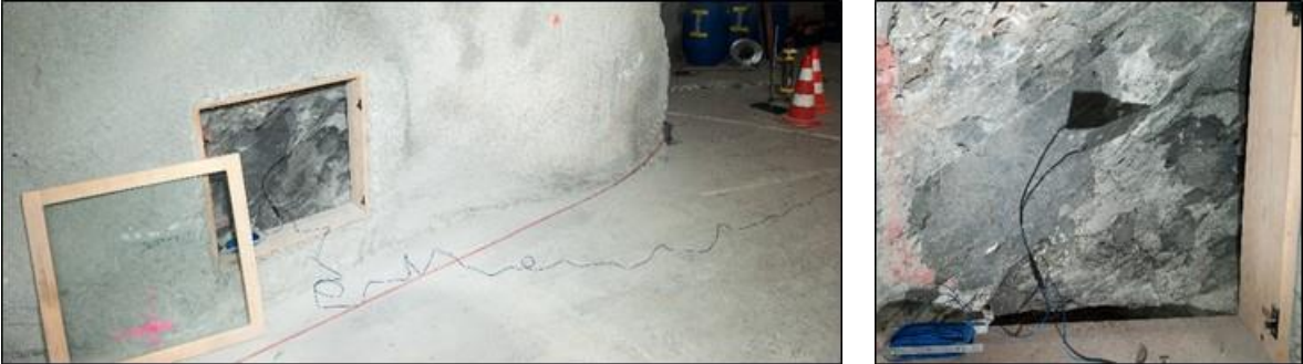
Figure 8.21 Left: the “geological windows” were used to connect the host rock (HE-D niche in the background), right: electrode installed in a crack
